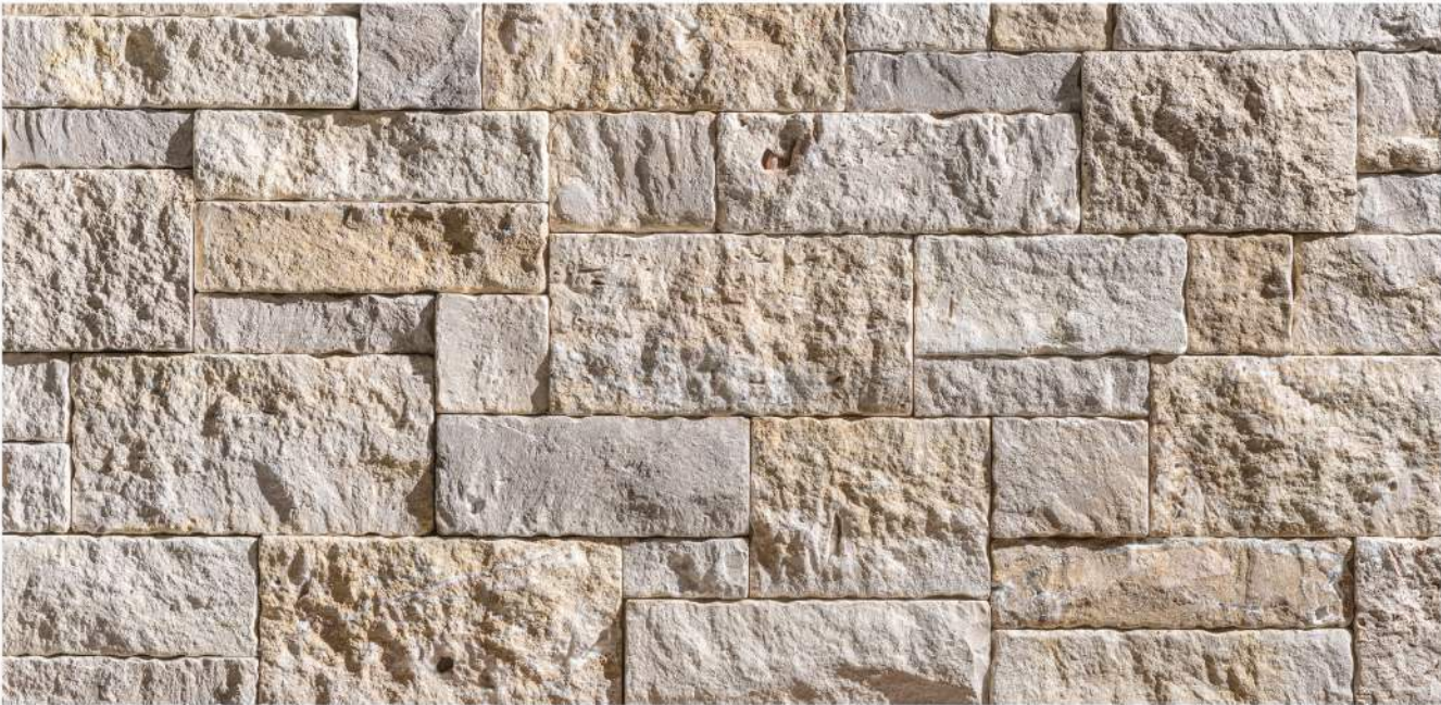
Photo Shows Dry-Stacked Installation
