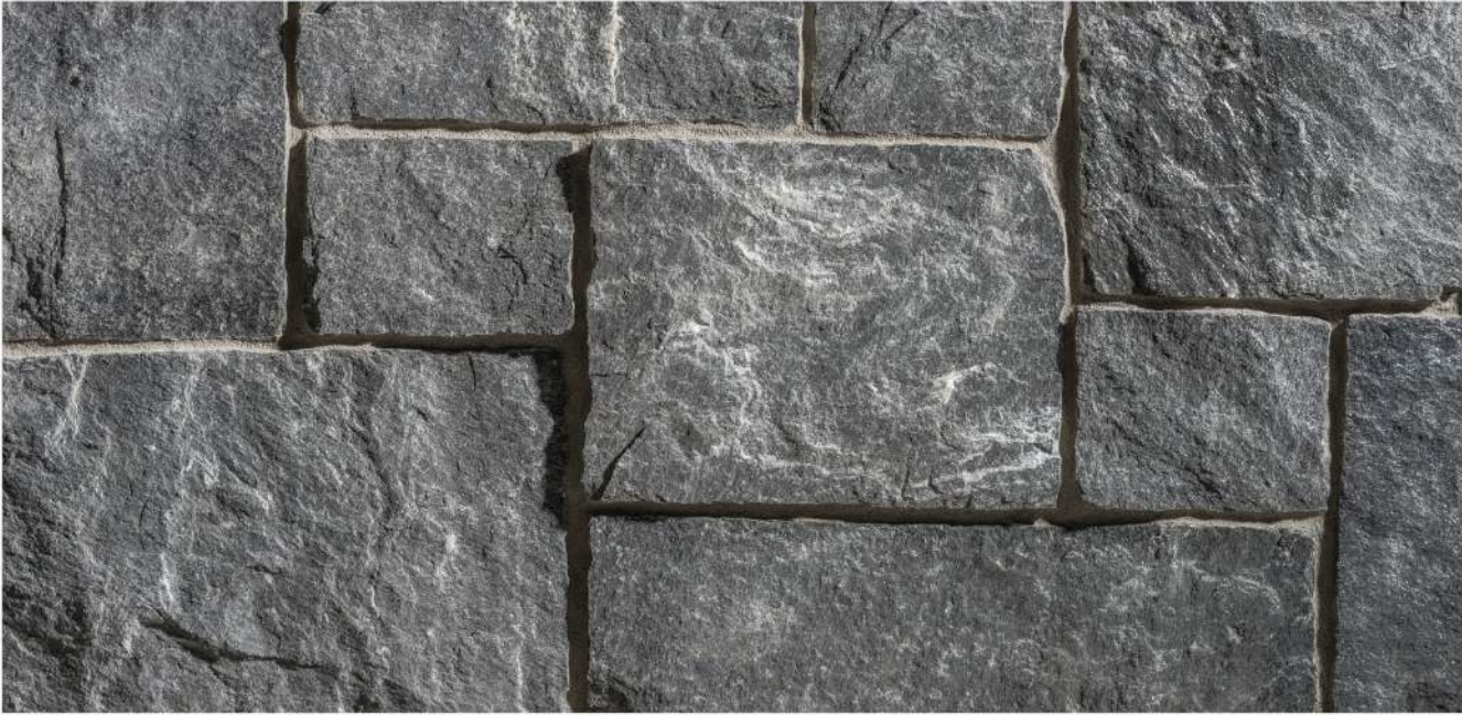
Photo Shows Installation With Mortar Joint
