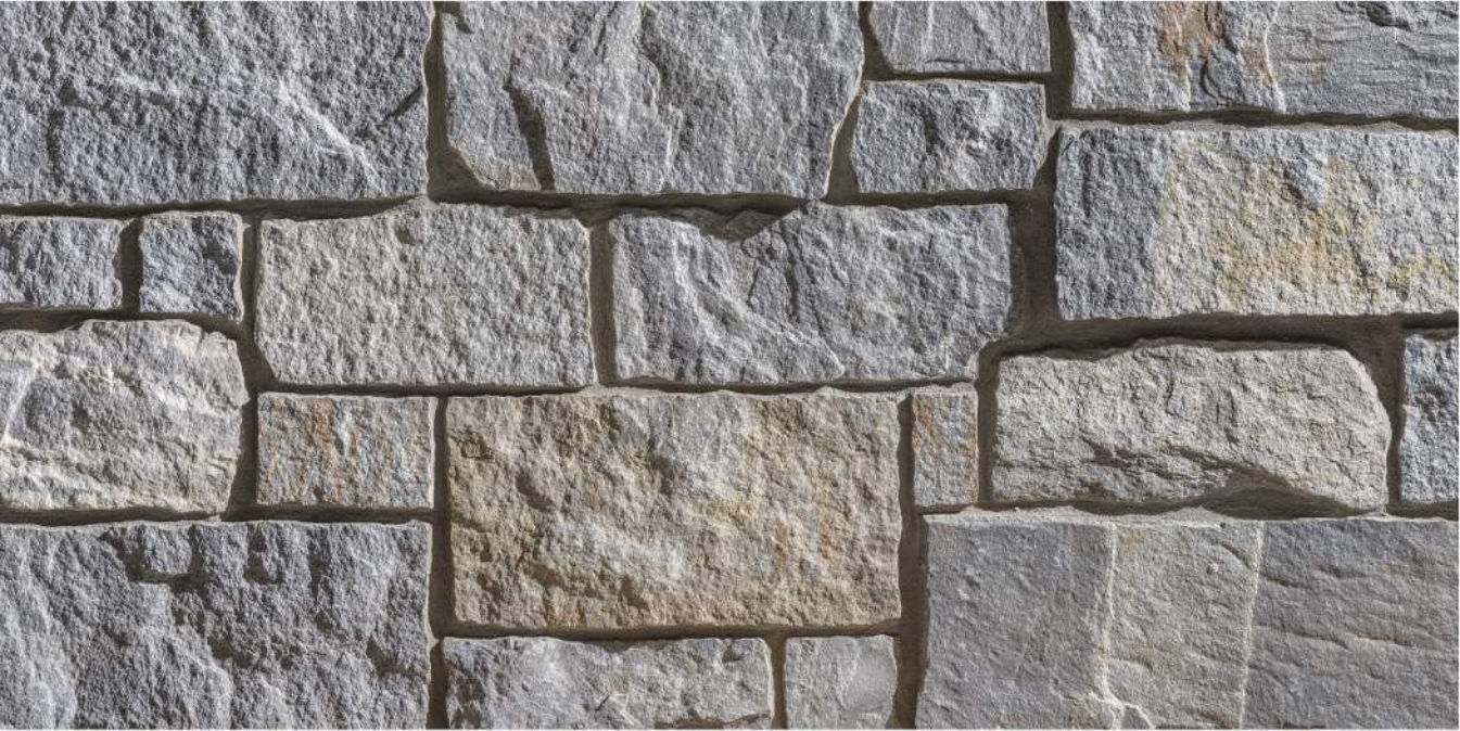
Photo Shows Installation With Mortar Joint
