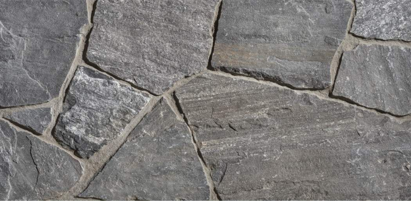
Photo Shows Installation With Mortar Joint
