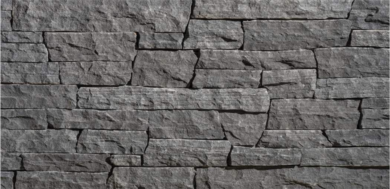
Photo Shows Dry-Stacked Installation
