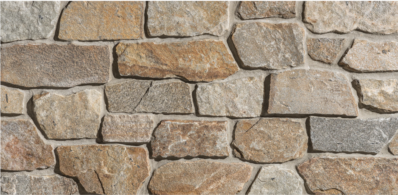
Photo Shows Installation With Mortar Joint
