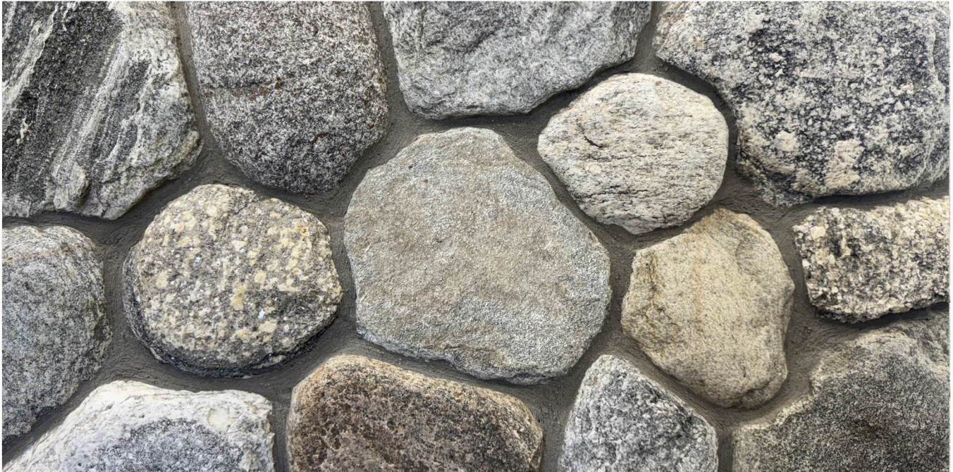
Photo Shows Installation With Mortar Joint
