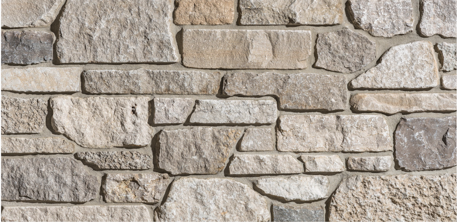
Photo Shows Installation With Mortar Joint
