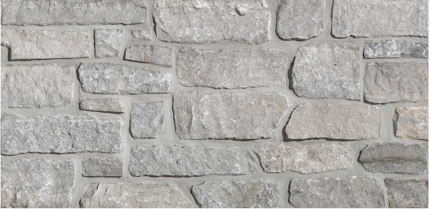
Photo Shows Installation With Mortar Joint
