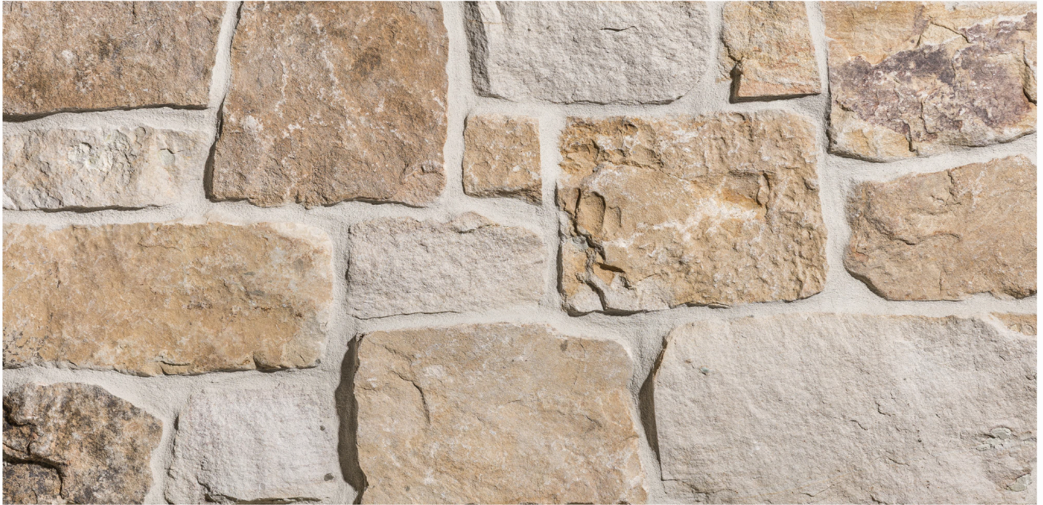
Photo Shows Installation With Mortar Joint
